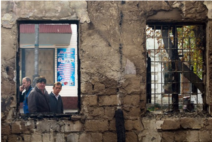
Local resident look at a destroyed building after recent shelling in the town of Popasna of Lugansk region on October 1, 2014. AFP PHOTO/ANATOLII BOIKO © AFP
